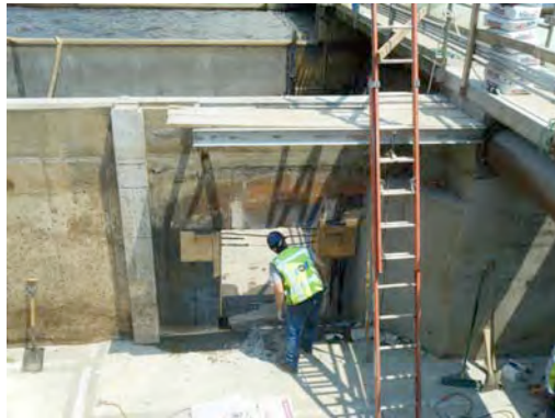
Rough opening cut into wall.
